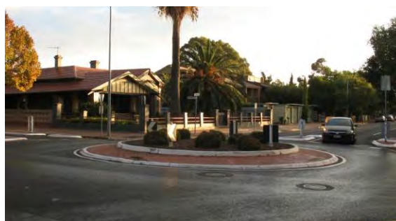
Figure 6.3 Small single-lane roundabout, Norwood, South Australia
